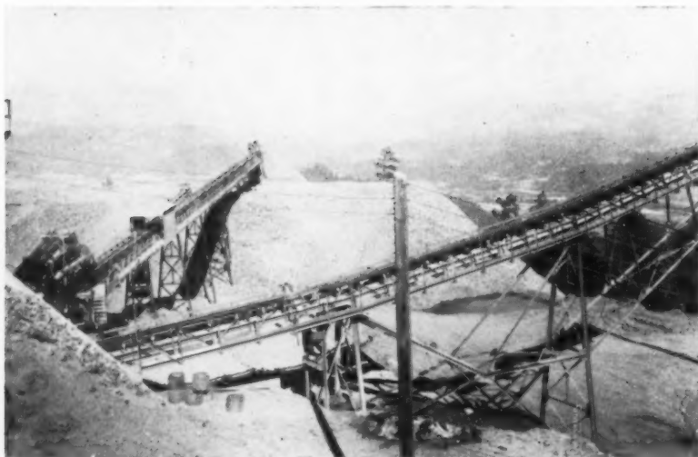
SCREENING PLANT has a wobbler feeder, jaw crusher, and a punched-plate screen. Conveyors send waste to reject pile (foreground) and ore to surge pile to right.
